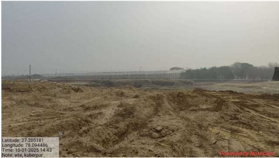
Pic-3- Land filling and levelling work in progress for WTE Plant
