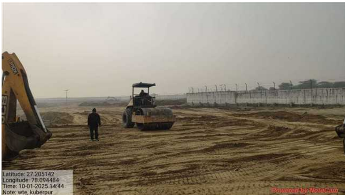
Pic-4- Land filling and levelling work in progress for WTE Plant
