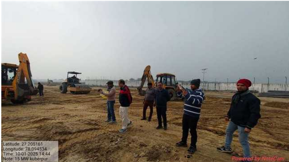
Pic-2- Land filling and levelling work in progress for WTE Plant
