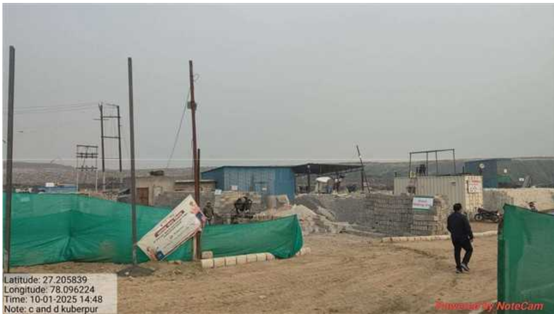
Pic-5- Functional C&D plant of Agra Nagra Nigam (20 TPD)
